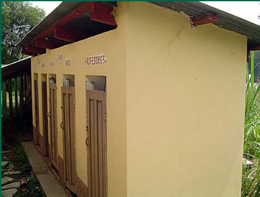
School Bathroom Construction
